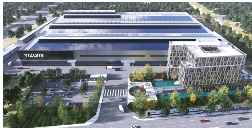
■ YIZUMI East China Production Base (In Construction)
